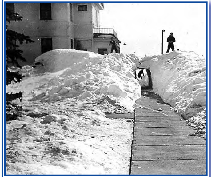
Sheyenne River Academy, tunnel from girls' dorm to main building.
