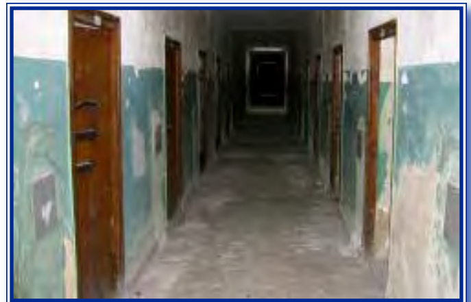
Hallway showing cell doors in one of the bunkers.
