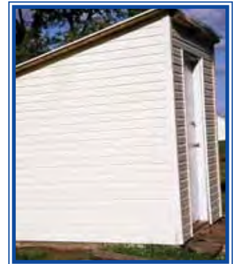
Completed root cellar with steel door, metal roof, vinyl siding and electrical lighting.
